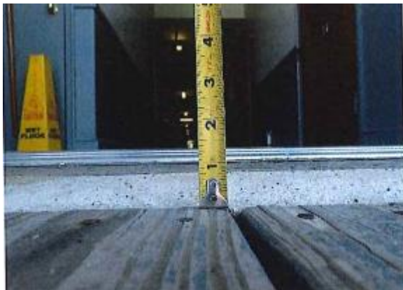
Figure 47: Gaps between planks and deteriorated, irregular concrete
