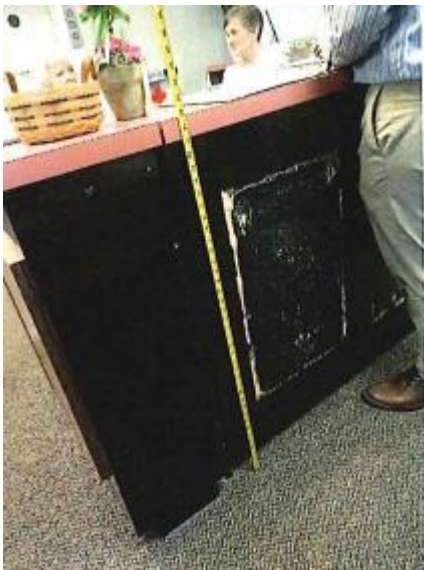
Figure 56: The COA Non-ADA compliant service counter
