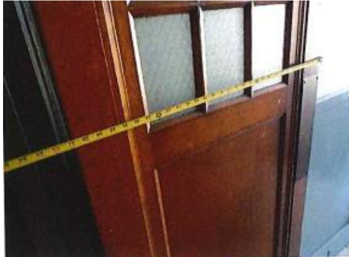
Figure 51: ADA non-compliant door width
