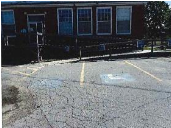
Figure 46: Switchback wood access ramp
