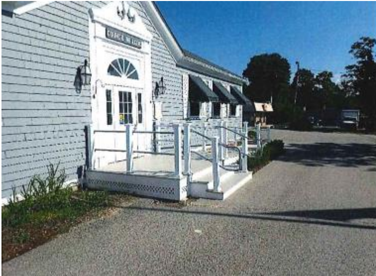
Figure 52: Pembroke Council on Aging
