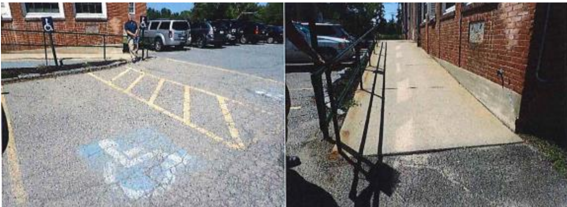
Figure 45: A straight run concrete access ramp leads to the building entrance.
