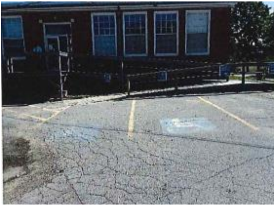
Figure 46: Switchback wood access ramp
