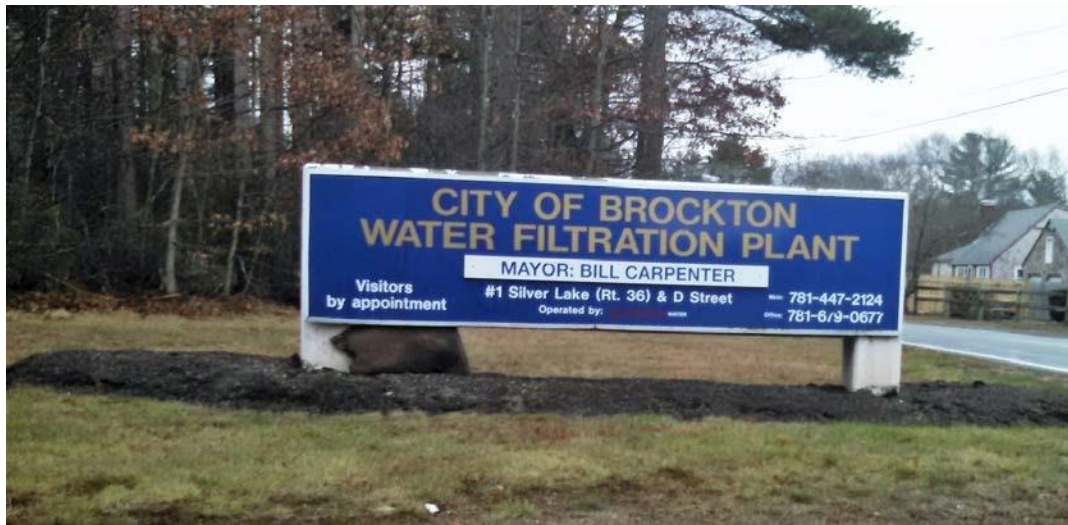
Figure 31: Brockton's water filtration plant in Pembroke
