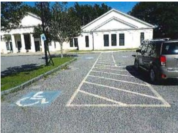
Figure 59: Pembroke Library Handicapped Parking Space
