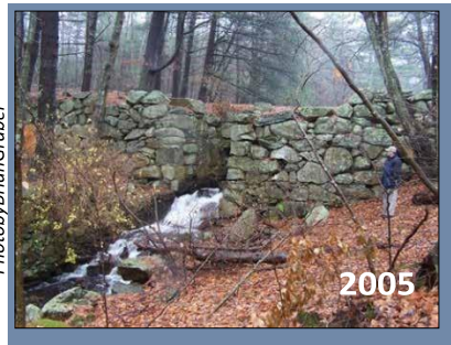
Figure 3. The Sawmill Pond Dam, built downstream of one of the bogs, altered the river's hydrology and blocked fish passage.
