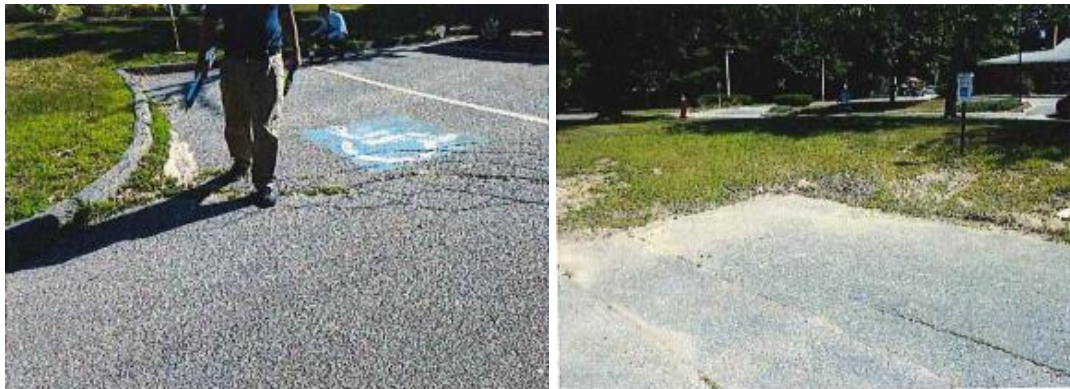
Figure 62: Pembroke Fire Station Handicapped Parking Space.
