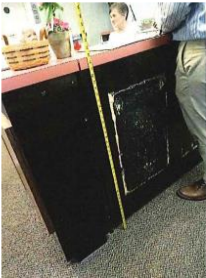
Figure 56: The COA Non-ADA compliant service counter
