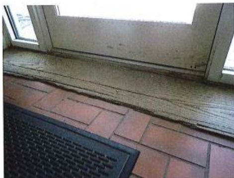
Figure 37: Town Hall Main (rear) entrance door and sill
