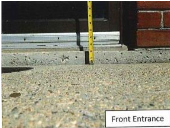
Figure 63: Pembroke Fire Station Main (front) Entrance
