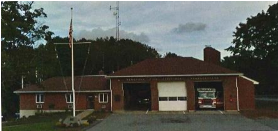
Figure 61: Pembroke Fire Station
