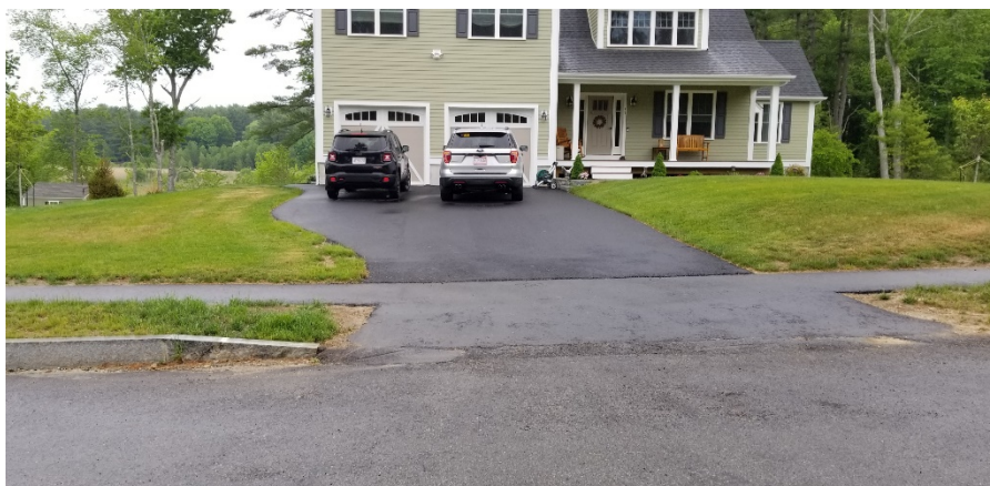
Driveway sloped to road, collection pipe is to the left of driveway
