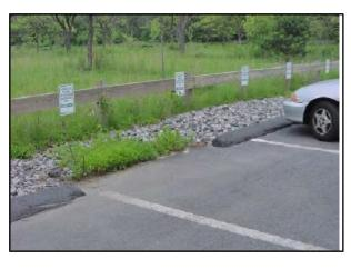
The picture to the left which is copied from the Stormwater Handbook shows a typical Vegetated Filter Strip which treats sheet flow and extends for the entire width of the parking area. The Drainage System Component shown on the submitted plans does not treat sheet flow; it treats a concentrated flow that has been conveyed to a single point. The Drainage System Component (as submitted) is not as wide as the area draining to the strip.
